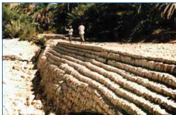
FIGURE 4.8 Diversion weir with stepped downstream face
