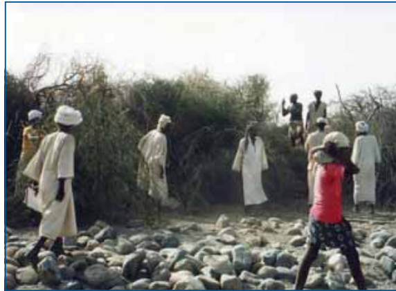
FIGURE 4.26 Bank protection using brushwood and boulders, Wadi Laba, Eritrea
