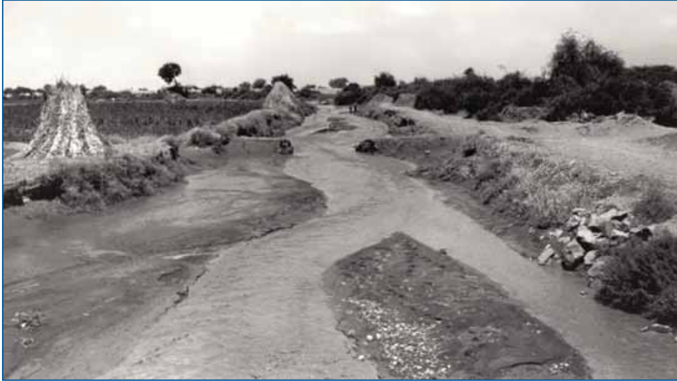
FIGURE 4.20 Traditional canal diversion bund, Wadi Zabid, Yemen
