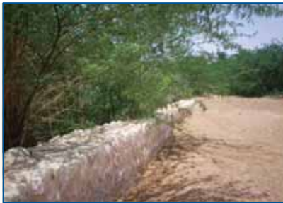
FIGURE 10.3 Recharge weir in Hadramawt, Yemen
